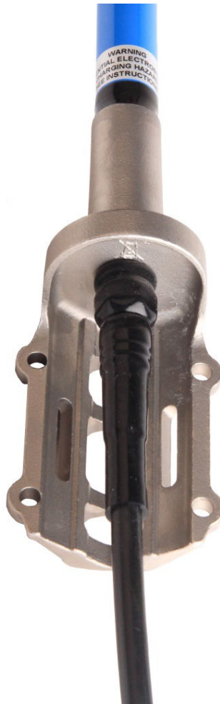
Figure 5: Installation of the “Cold shrink PST B3 4.5/125/24.2” on the connection is complete.
